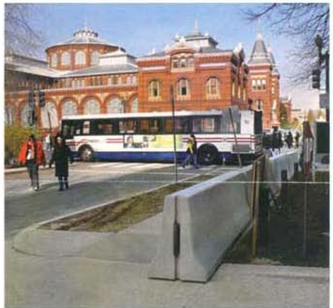
Smith-Midland Corp. installed 17,000 sf of concrete barriers in Washington, D.C., for the Inauguration.
